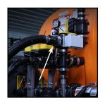
**13)** Power applicator pump on and move the 3-way valve on top of pump in the discharge position.
